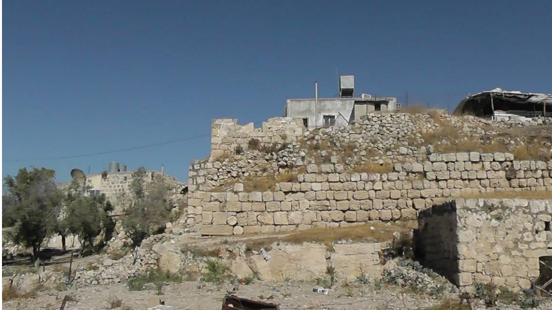
Al-Burj – house built alongside and atop ancient remains
